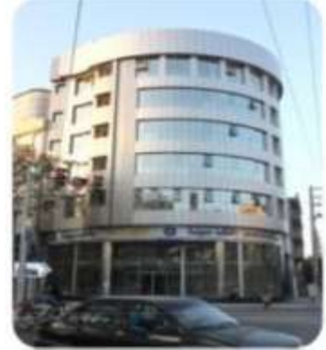
Sina Commercial-Administrative Complex in Sari
