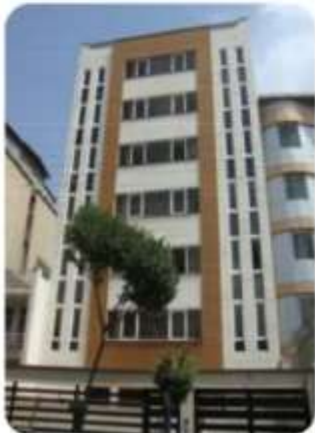
Pars Sina Administrative Complex
